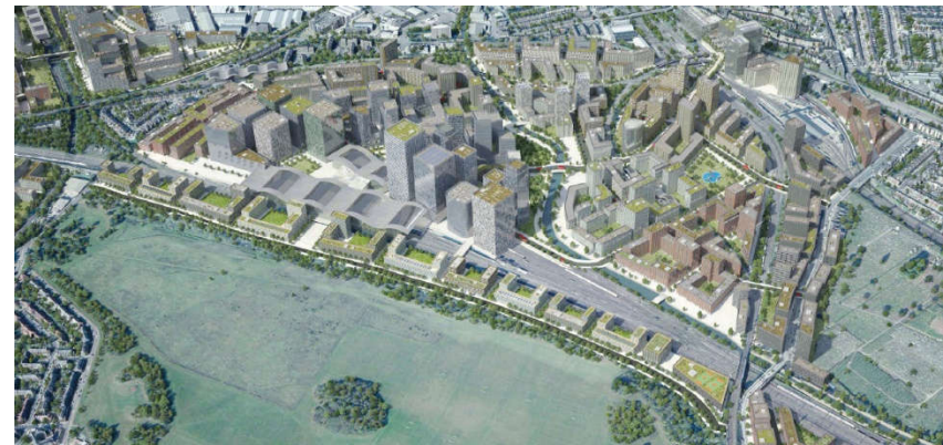
Aerial view of Old Oak indicative development proposals. Source: Environmental Target Setting Study, Old Oak and Park Royal Development Corporation, 2017 .
