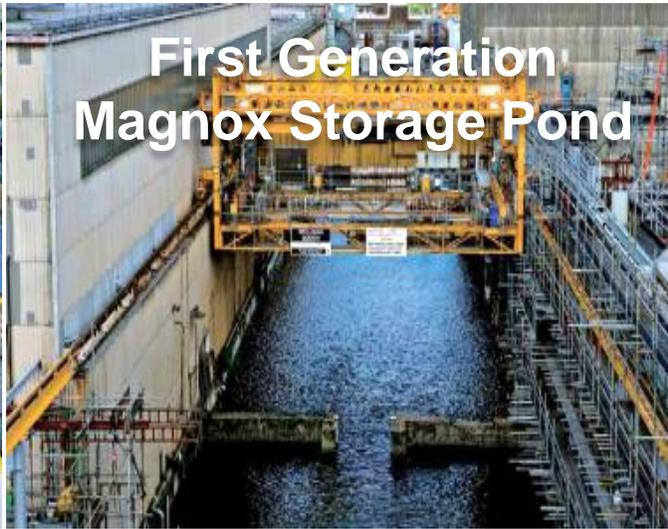
Constructed in 1950s and 1960s to store Magnox fuel for reprocessing. Waste consists of sludge, fuel, intermediate and low level waste.
