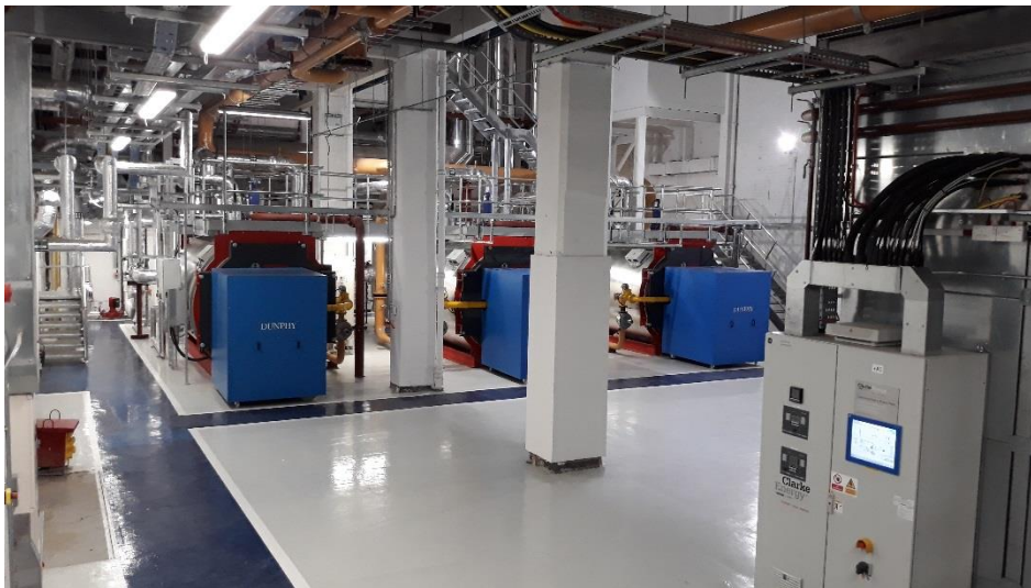
Figure 1 - The new 24MW boiler plant in the refurbished energy centre.
