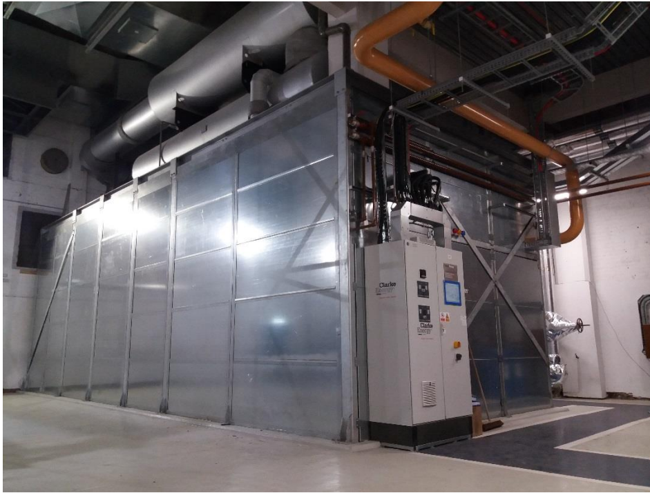
Figure 2 – the newly installed Combined Heat and Power 3.3MW engine in its acoustic enclosure
